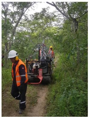
Photo 1: Transporting components of the drill rig to site using motorised trolleys along existing tracks
