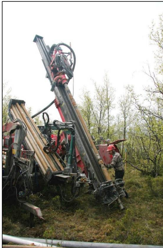
RC drill rig on site at Viscaria
